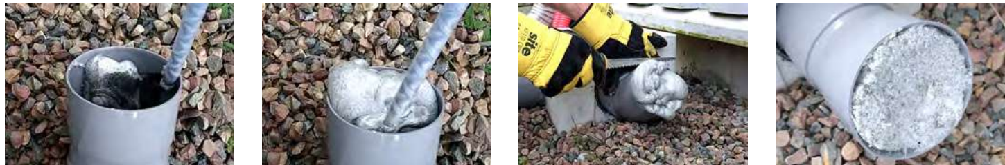
Seal PVC pipes with PFP Foam – in under 5 minutes
