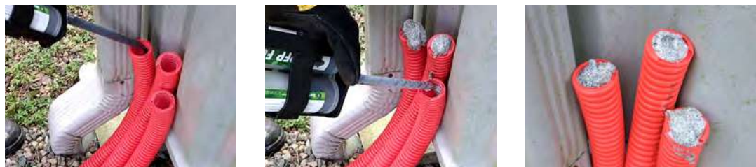
Fill technical ducts with PFP Foam
