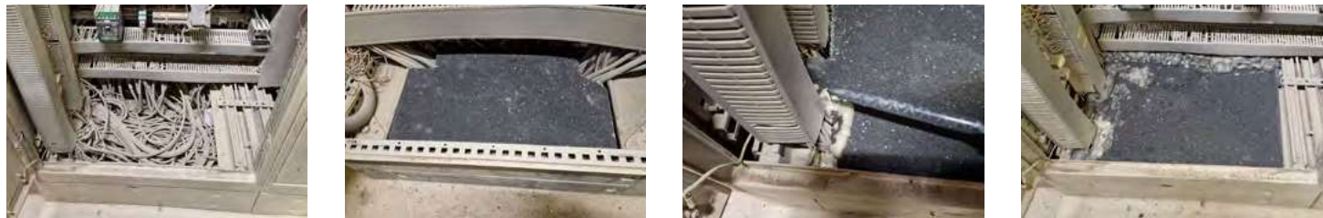
Protect an electrical cabinet using a rodent-proof panel and PFP Foam
